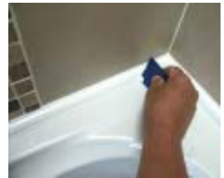
Change to fine nozzle - Seal in top and bottom of profile with silicon - Fit End Caps - Use Fugi to remove excess silicone - Leave to set 4 hours
