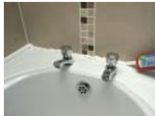
Clean Profile - Fit the long length 1st - Add generous silicone with large nozzle - Fit profile and remove excess with Fugi - Now fit end pieces
