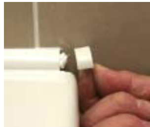
Change to fine nozzle - Seal in top and bottom of profile with silicon - Fit End Caps - Use Fugi to remove excess silicone - Leave to set 4 hours
