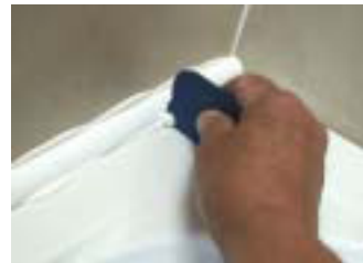
Clean Profile - Fit the long length 1st - Add generous silicone with large nozzle - Fit profile and remove excess with Fugi - Now fit end pieces
