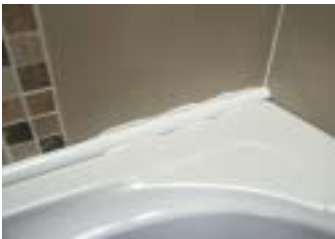
Clean Profile - Fit the long length 1st - Add generous silicone with large nozzle - Fit profile and remove excess with Fugi - Now fit end pieces
