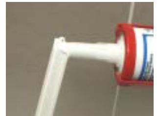
Clean Profile - Fit the long length 1st - Add generous silicone with large nozzle - Fit profile and remove excess with Fugi - Now fit end pieces
