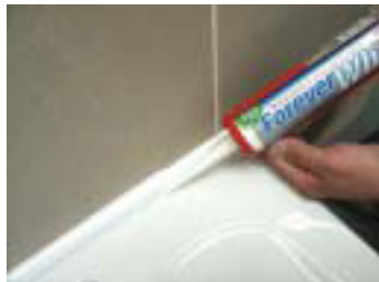
Change to fine nozzle - Seal in top and bottom of profile with silicon - Fit End Caps - Use Fugi to remove excess silicone - Leave to set 4 hours
